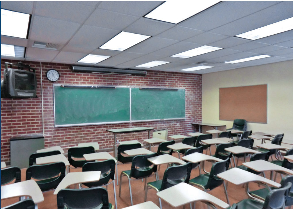
Post-retrofit luminaires at Laney College in Oakland, CA.
